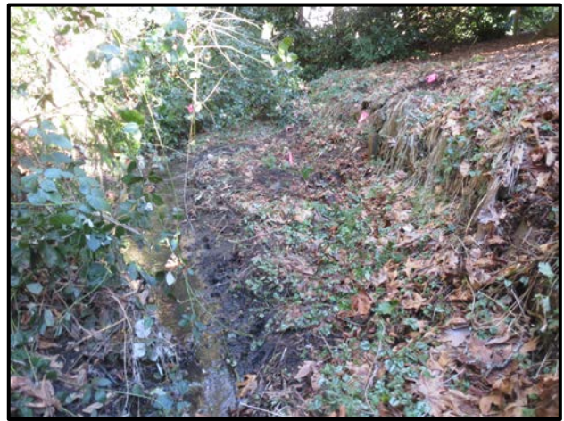
Figure 5: Facing North Towards Wetland A
